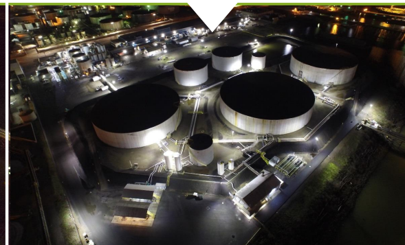
After PEC Installation
